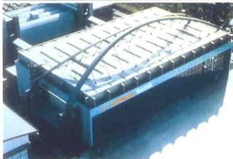
▲ Jumbo aircraft hangar, Hamburg Airport
